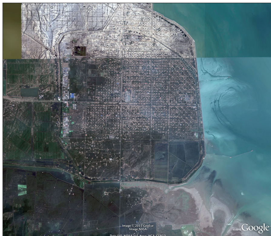
Figure 1: GEO-EYE satellite image of the Yellow River (Huanghe) delta. Each year 33.6 Mt of crude oil are extracted from the delta. The Gudong Seawall, built 1985–1988 to protect the oil fields from inundation, is 10 m thick at its top and 38 m at its bottom. The oil rigs are laid out on a grid pattern. The field is presently below sea level by 1 to 2 m, protected from the sea by the Seawall. Image from Google Earth Pro; pixel resolution is ~1 m.
